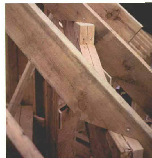
Method #1: raised block. Nailing triangular blocks on the sloping, angled headers created a level surface to seat the rafters on. But this required a deep heel cut on the bird's mouth and weakened the rafter overhang.
