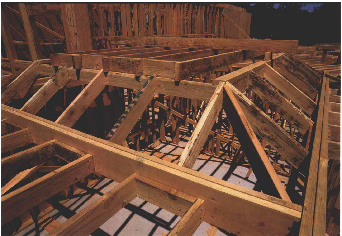
A topless hip. Once the soffit is in place, framing for the coffer itself is like a hip roof with the top removed. Pressure blocks are nailed between framing members on either side of the doubled carrier box; the blocks prevent the framing from twisting as it dries.
