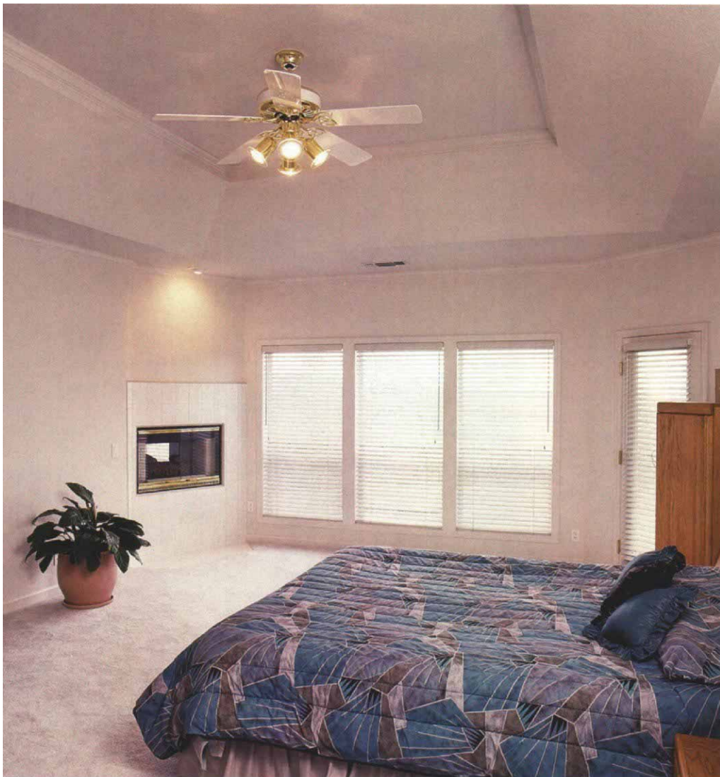
One big coffer. Soffits girdle this bedroom to support angled coffer framing. A single, recessed ceiling coffer is the result. Photo by Scot Zimmerman.
