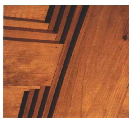
Adding up the ribs. Stepped layers of 1x stock in various widths form the ribs of the coffer. Transverse ribs are slightly wider and one layer thicker than lengthwise ribs.
