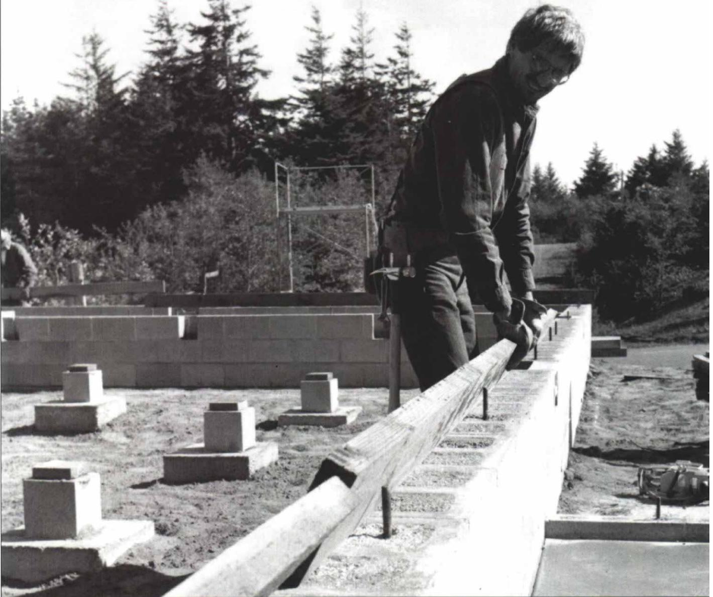
**Straightening bolts and scattering sills.** Bent anchor bolts can be straightened easily by levering them into plumb with a length of  $\frac{3}{4}$ -in. pipe (below). That done, it's time to set the sill stock roughly in place on the foundation prior to marking and cutting it (above).
