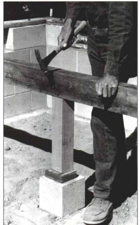
**Bracing and splicing the girders.** Joints between lengths of girder should fall over a post and be secured with straps or gussets. If the posts are more than 3 ft. tall, they should be braced to increase the stability of the system.
