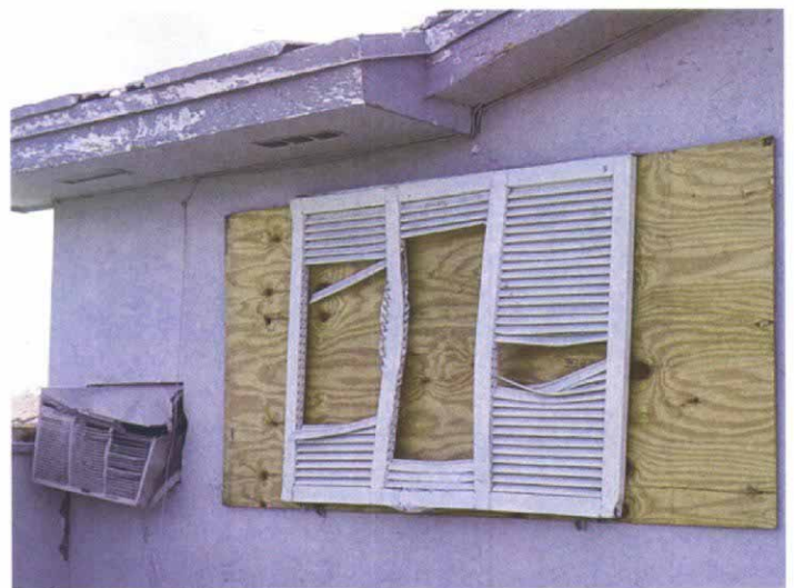
Useless shutters. Plywood now covers the window smashed by the roof tiles that went through this aluminum louvered shutter.
