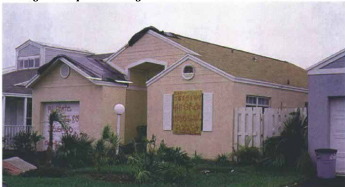
Useless shutters. Plywood now covers the window smashed by the roof tiles that went through this aluminum louvered shutter.
