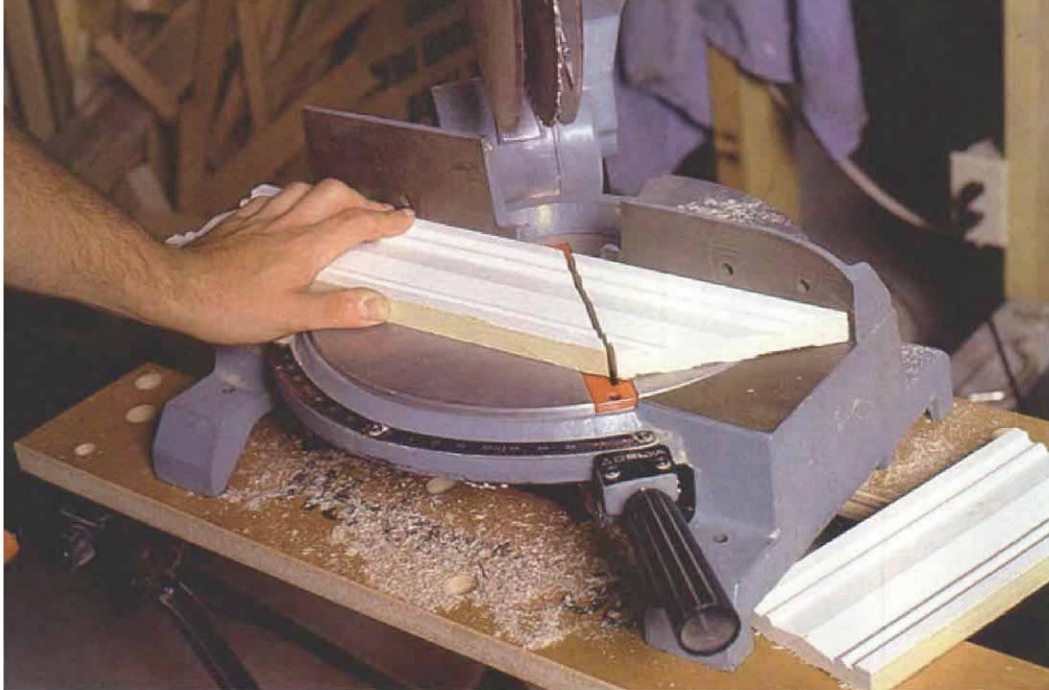
Cutting the corner-block components. Two 45° cuts make a triangle, and four of these triangles make a square corner block. The full width of the casing was used for the end corner blocks.
