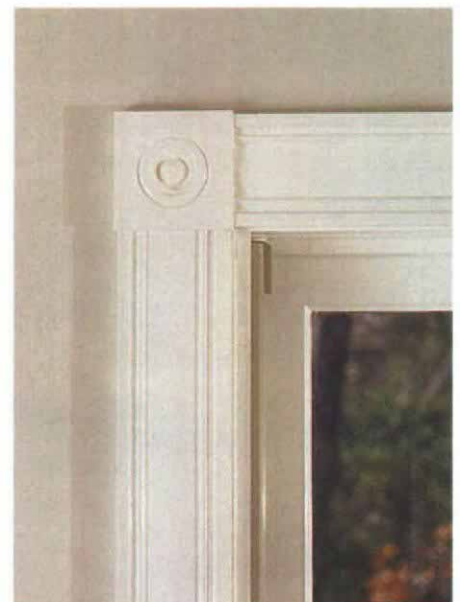
Interior detail. Custom-milled corner blocks and casing inside the house inspired the design for the front-door exterior trim.
