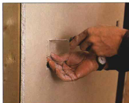
Saw and slice. Another way to cut holes for outlets is to first hang the drywall right over the boxes. Then use a drywall saw to cut around the interior of the box. Remove the waste and enlarge the opening with a utility knife.
