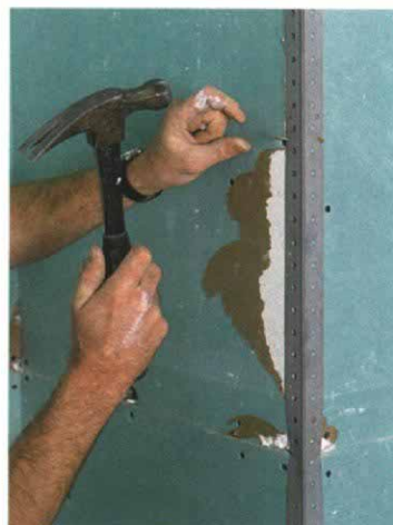
Outside corners. Metal corner bead protects the drywall at a vulnerable location and makes it easy to get a crisp, finished edge that runs straight from base to crown.
