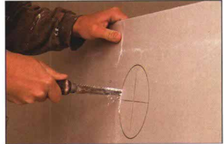
Twirl and cut. You can mark circular cutouts with a compass made from a screw and a piece of the paper used to bind pairs of drywall sheets at their ends. Plunge a drywall saw through the face paper to make your cut.
