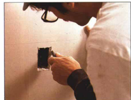
Saw and slice. Another way to cut holes for outlets is to first hang the drywall right over the boxes. Then use a drywall saw to cut around the interior of the box. Remove the waste and enlarge the opening with a utility knife.
