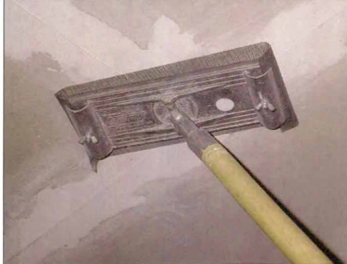
Labor saver. A pole sander brings ceilings closer and keeps drywall dust at arm's length.
