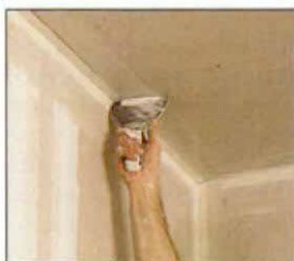
Taping inside corners. After knifing a bedding coat onto the wall and ceiling, drywall taper Brian Henderson pushes a folded strip of paper tape into the corner (above). Then he sets the tape into the compound with a tapping knife and at the same time removes the excess joint compound.
