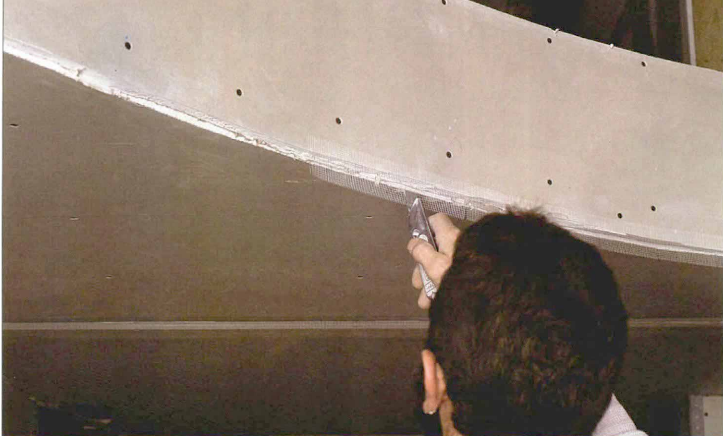
Taping a curve. The corner is covered with an adhesive-backed mesh, which is cut into segments to lie flat on the ceiling (above). A strip of metal-reinforced corner tape is then sliced in half (below left) and bedded in setting-type compound (below right). The bottom of the tape extends \frac{1}{16} in. past the corner. This protruding metal edge guides the knife as the space behind it gets filled in with joint compound.
