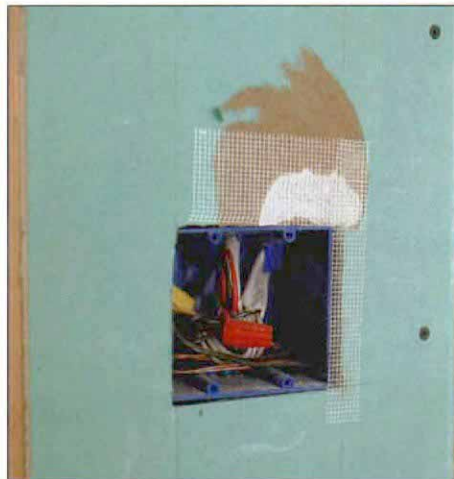
Patching and filling. Use mesh tape over cavities and gaps that need patching (photo above left). Then fill them with setting compound. You can also use setting compound to fill the gaps between fiberglass shower stalls and the adjacent drywall (photo above right). Once the filler sets up, the seam between it and the surrounding drywall should be taped like a buttjoint.
