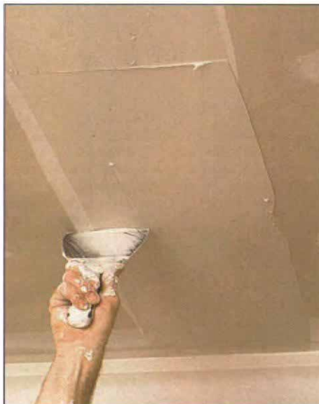
Top coat and feathering. Finish coats of joint compound are applied with a wide knife or trowel (above left). Then the ridges along the edges are taken out with a taping knife held at a slight angle (above right). In his left hand Henderson holds a metal hawk—a palette for holding joint compound. Its rim makes a handy place for cleaning the edges of drywall knives and trowels.
