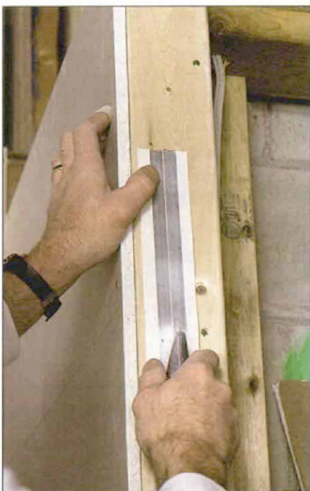
Taping a curve. The corner is covered with an adhesive-backed mesh, which is cut into segments to lie flat on the ceiling (above). A strip of metal-reinforced corner tape is then sliced in half (below left) and bedded in setting-type compound (below right). The bottom of the tape extends \frac{1}{16} in. past the corner. This protruding metal edge guides the knife as the space behind it gets filled in with joint compound.
