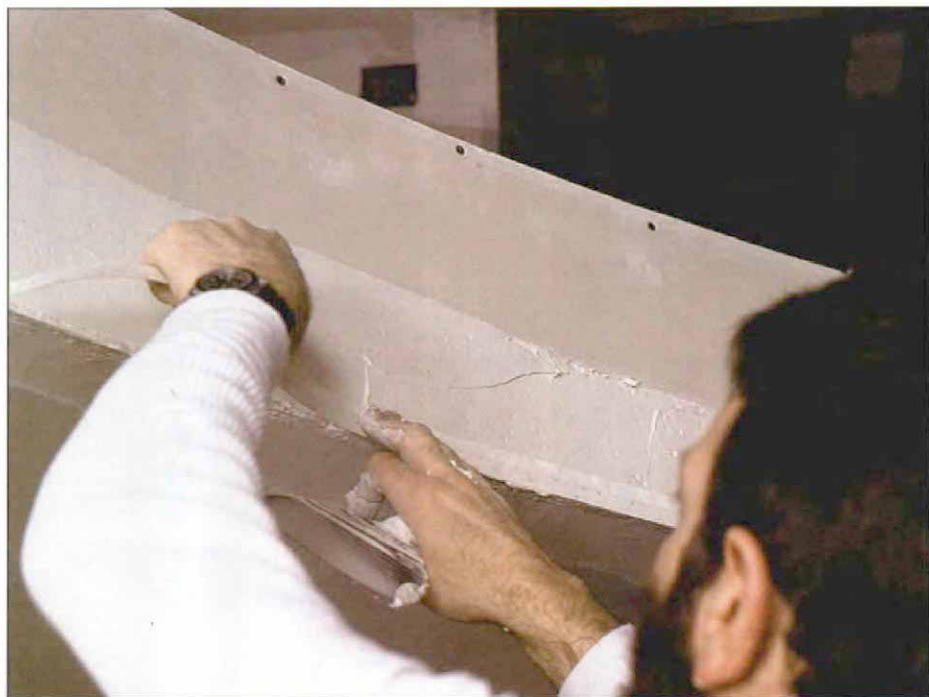
Taping a curve. The corner is covered with an adhesive-backed mesh, which is cut into segments to lie flat on the ceiling (above). A strip of metal-reinforced corner tape is then sliced in half (below left) and bedded in setting-type compound (below right). The bottom of the tape extends \frac{1}{16} in. past the corner. This protruding metal edge guides the knife as the space behind it gets filled in with joint compound.
