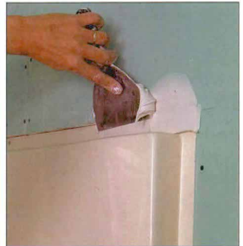
Patching and filling. Use mesh tape over cavities and gaps that need patching (photo above left). Then fill them with setting compound. You can also use setting compound to fill the gaps between fiberglass shower stalls and the adjacent drywall (photo above right). Once the filler sets up, the seam between it and the surrounding drywall should be taped like a buttjoint.
