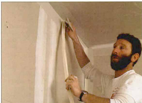
Taping inside corners. After knifing a bedding coat onto the wall and ceiling, drywall taper Brian Henderson pushes a folded strip of paper tape into the corner (above). Then he sets the tape into the compound with a tapping knife and at the same time removes the excess joint compound.
