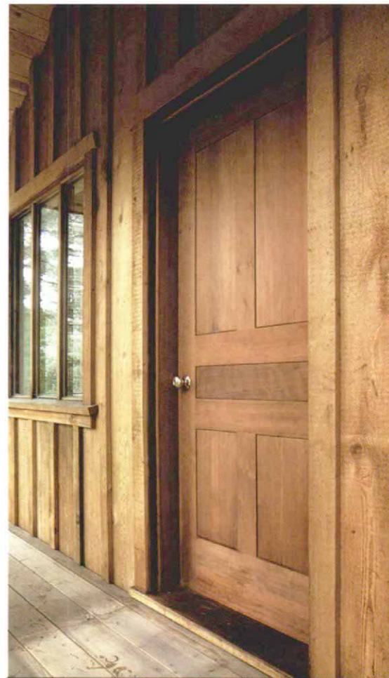
All it takes are butt joints. Cherry panels floating in a redwood frame warm a room otherwise dominated by a gray carpet and white walls (photo above). The author made the doors on site to match the trim details found throughout the house. The panels in the exterior door (photo below) are narrower, which reduces seasonal swelling and shrinking.
