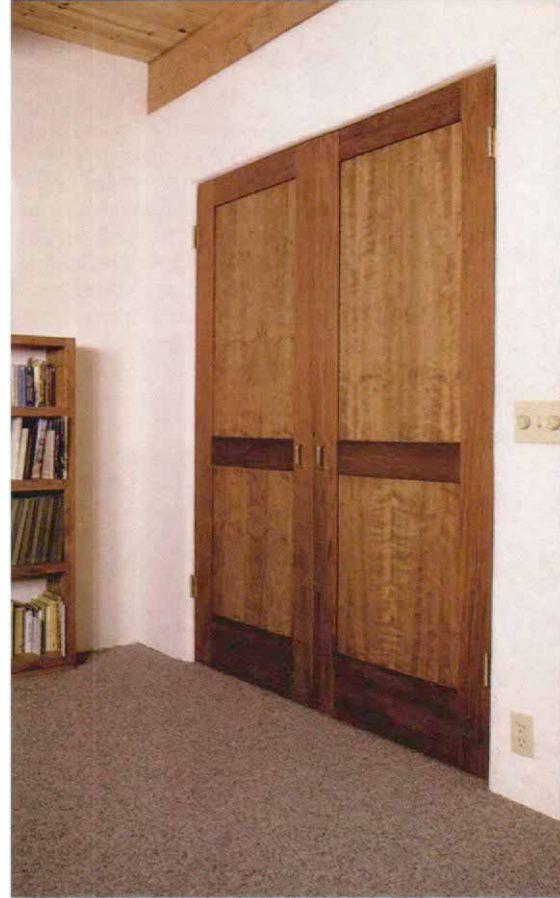
All it takes are butt joints. Cherry panels floating in a redwood frame warm a room otherwise dominated by a gray carpet and white walls (photo above). The author made the doors on site to match the trim details found throughout the house. The panels in the exterior door (photo below) are narrower, which reduces seasonal swelling and shrinking.
