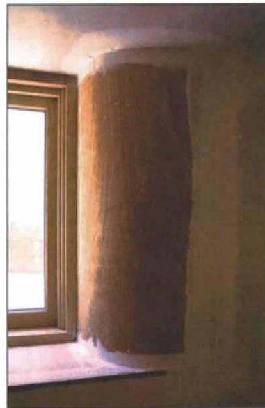
**Brightening the basement.** Bending plywood opens up window returns in furred-out walls. The window frame was built up with two layers of conventional plywood, creating pockets that hold the drywall sill and ceiling and the bending plywood returns.
