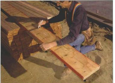
Skip the tape. When cutting short lengths of blocking from a long 2x, there's no need to measure and square each block separately. Instead, the author uses his framing square to mark off blocks quickly. He aligns the end of the 2x with the correct measurement on the inside of the square's blade, uses the tongue to mark a square line across the 2x and then moves the square along the 2x to repeat the process.
