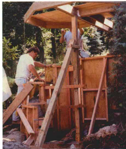
Plumbing the forms. Plumb lines at the deck corners help locate the foundation forms.
