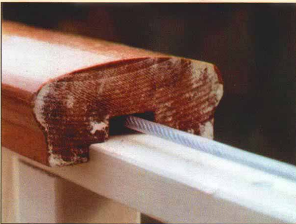
Handrail conceals cable. This cedar handrail was grooved to hide the cable. Once the cable was tight, the handrail and a corresponding rail at the bottom of each section were fastened to the newels with galvanized 16d finish nails.
