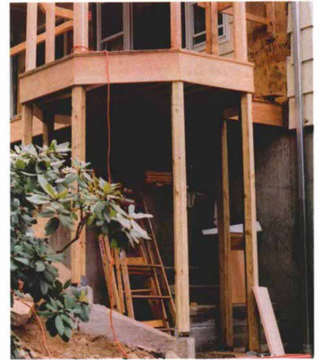
Beveled supports. Posts were milled to continue the octagon down to the retaining wall.
