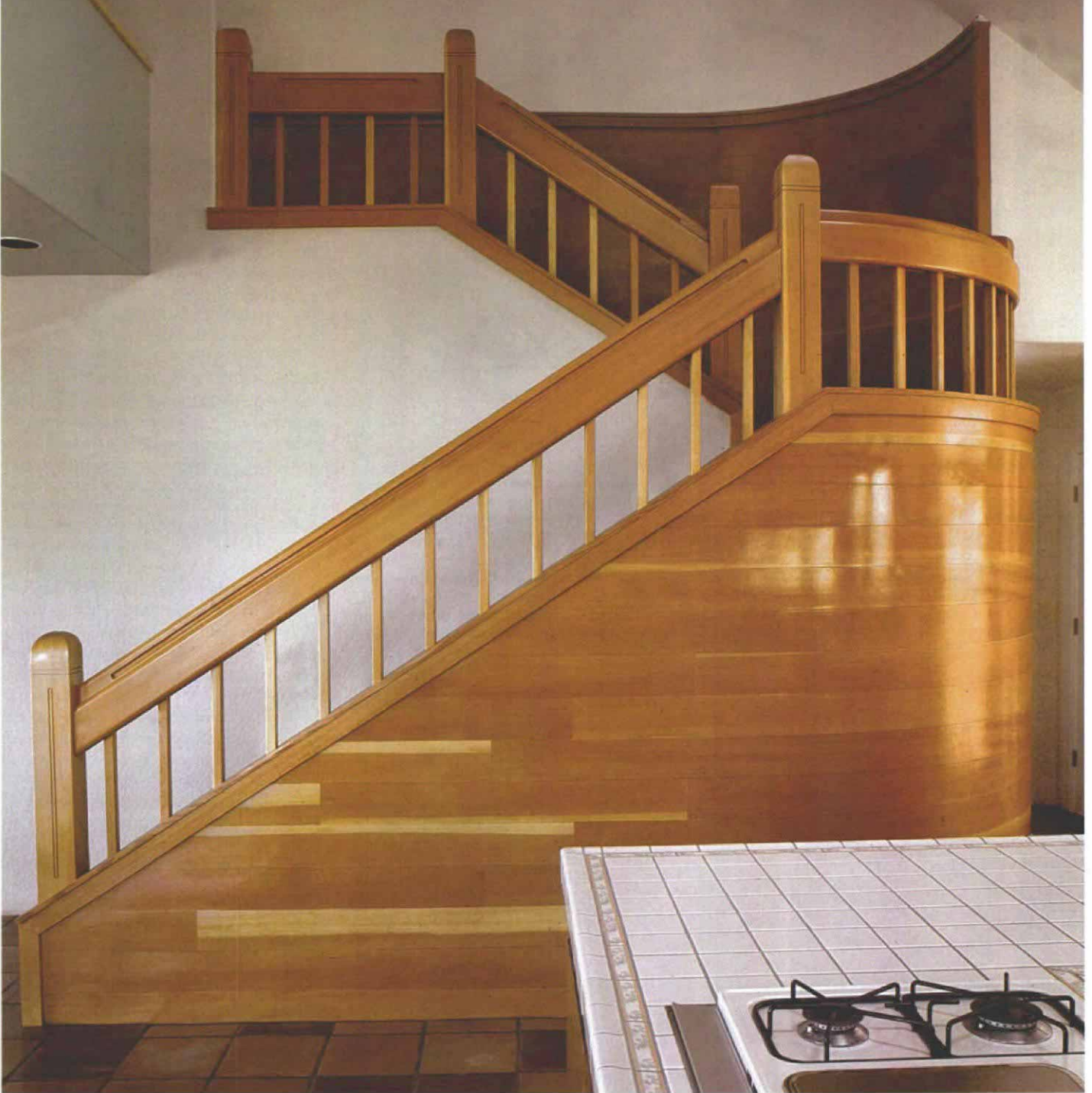
Curved fir. A unique curved stair, which draws attention to itself for its sheer size and complexity, fits neatly into the overall plan of the house.
