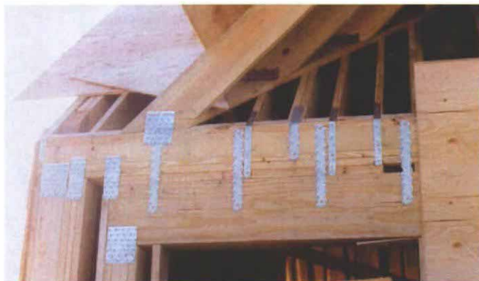
Hurricane straps. Typical of the detailing throughout the house, every rafter was fastened to the walls with galvanized metal straps.
