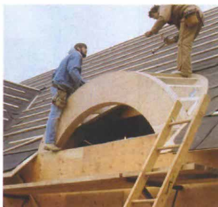
Plywood header. The header for the arch top kitchen window is made of seven layers of \frac{3}{4} -in. plywood cut to fit the window's curves.
