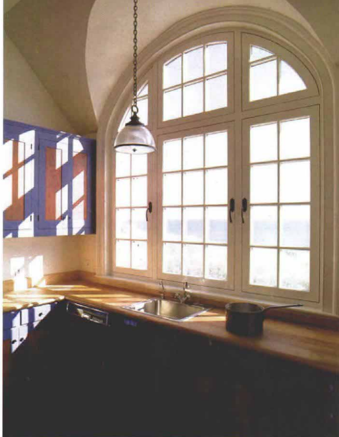
Curved cornice in an eyebrow dormer. The focal point of the house's ocean-side facade is the large, 40-lite kitchen window seen here from the interior (left) and the exterior (right). The curved five-piece exterior cornice terminates in bracketed water tables.
