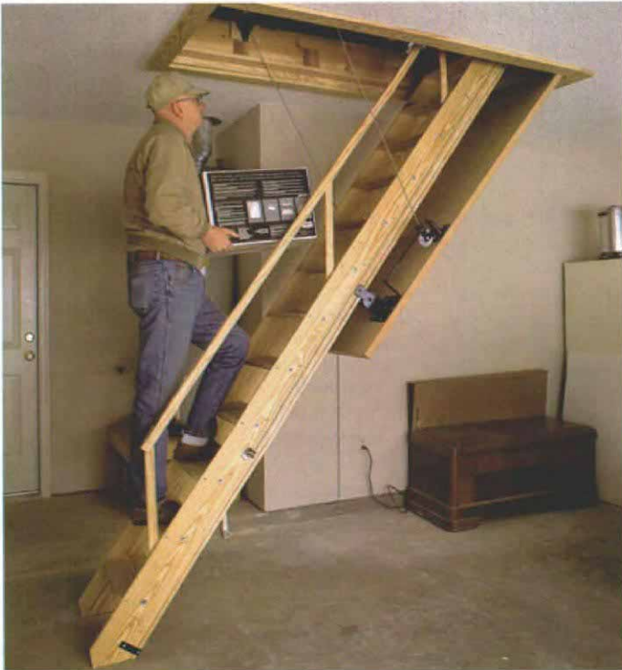
Sliding stairway. Disappearing stairways are concealed by a spring-loaded ceiling door. Here, the author walks up a sliding stairway made by Bessler with an angle of incline close to that of a permanent stairway.
