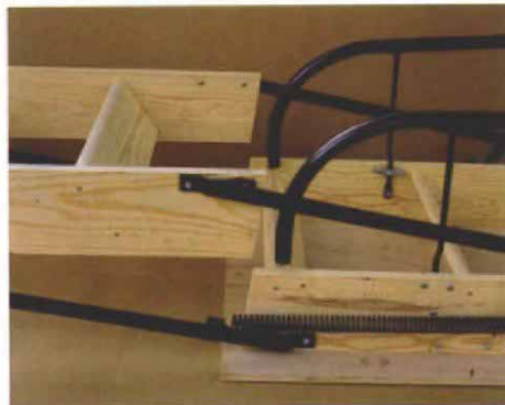
Hinged sections. Hollywood Stairways have ladderlike sections that are hinged like a parallel ruler. When opened fully the sections butt at their ends. On the right you can see the steel-tube handrails. When the stairway is opened fully, the handrails project 18 in. above the attic floor.
