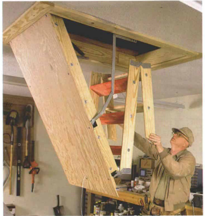
Folding stairway. Ladderlike sections are hinged like an accordion to the ceiling-mounted door. On this model, made by American Stairways, the treads are painted with bright-colored, rubberized paint.
