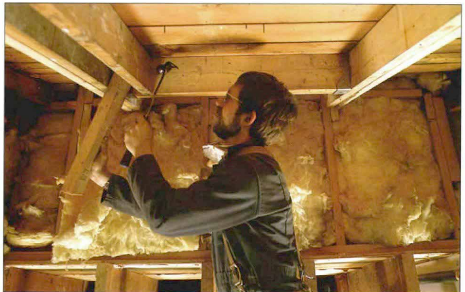
Establishing the well width. Using a short section of a 2x4, the author wedges a rafter in place and toenails it to the header. He'll add a metal hanger later to help carry the roof loads.
