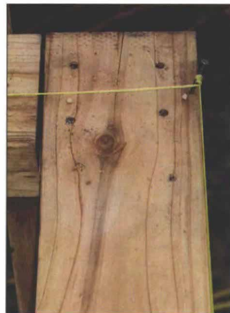
Using a line without blocks. You can tell if a wall is straight by stringing a tight line from one end of a top plate to another. A nail is bent flush with the outside plane of the wall, and another nail is tacked to the opposite corner.
