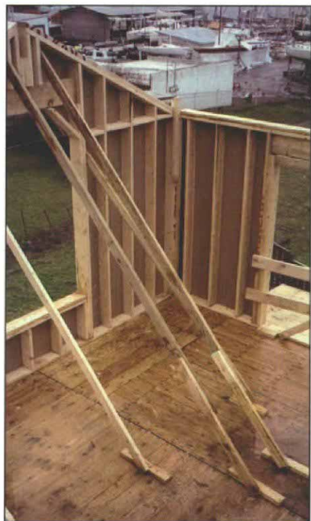
Line braces hold walls straight. This gable end is straightened and held straight with 2x4 line braces. Note the line running along the blocking. The top of each brace is nailed to the wall just below the plate. The bottom of each brace is left square so that it can be pushed forward with a crowbar, just like a racking brace. When the wall is straight, the line braces are nailed to cleats. The cleats are spiked to the floor joists, not just to the plywood deck.
