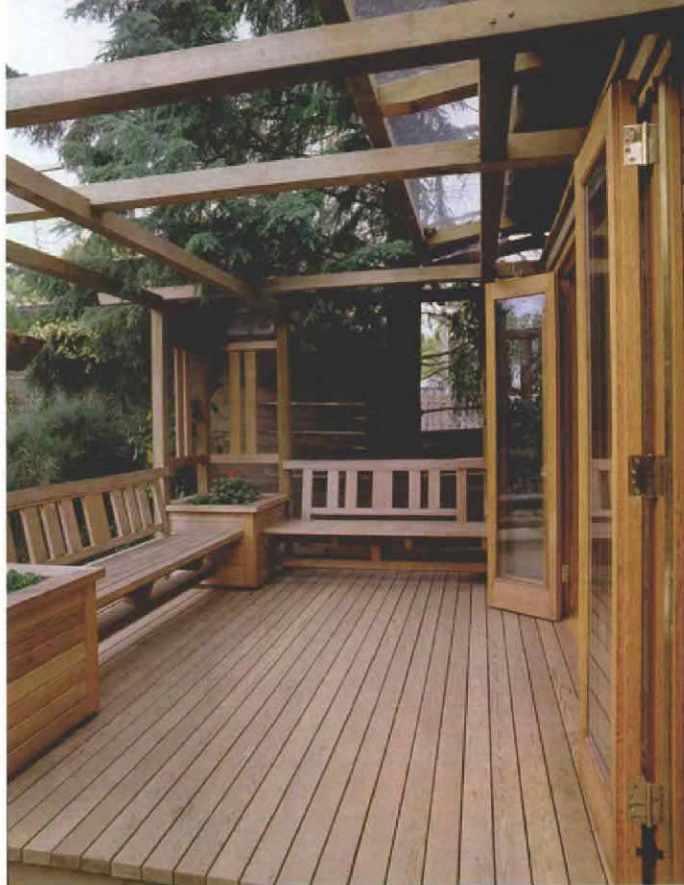
Partly in, partly out. Built-in benches and planters at the corners make a boundary around the sides of the deck, and the spare trellis overhead implies a ceiling. The planters brace the posts at the corners.
