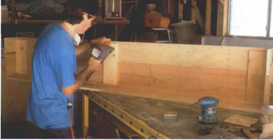
Frieze box has plywood upper half and solid-wood lower half. This part of the mantel top will be capped with a shelf and covered with trim, and only the solid-oak lower half will be exposed. The plywood and the solid wood are biscuited together, and blocking supports the joints.
