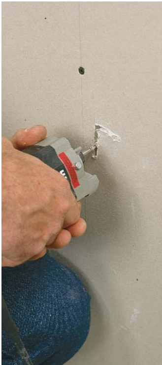
Any trimmer can be used to cut drywall. Porter-Cable takes the same motor that's on its 7310 laminate trimmer, packages it with some drywall cutout bits and sells it as a 7399 Drywall Cutout Tool.
