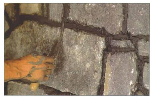
**Smooth the mortar to get the look you want.** After filling the joint with mortar, smooth over it with a pointing trowel to get the joint to the desired smoothness. For a slightly recessed joint that reveals the shape of the stones better, scrape the tip of the pointer along the inside edge of the stones.
