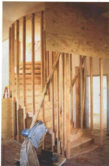
**Inside the staircase.** Assembly of the stair (far left) starts with a plywood and stud armature. A pair of plywood patterns defines the plan of the stair (drawing below). Pairs of studs (left) carry 2x12 cross ties that serve as risers for the stair. Blue tape (below) shows where the cuts were made to remove everything that's not part of the finished stair.
