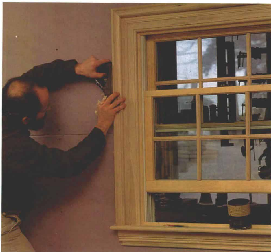
Plane the edges even. It's possible that the outside edges of all of the built-up moldings of a mitered casing won't be perfectly flush after they're nailed on. A couple of passes with a bench plane makes a flat surface. The last few inches at the bottom are cleaned up with a sharp chisel.
