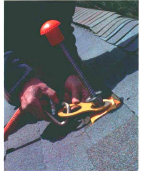
It won't open accidentally. This self-locking snap hook, also called a carabiner, is used to attach a lifeline to an anchor and won't open unless two actions are executed.
