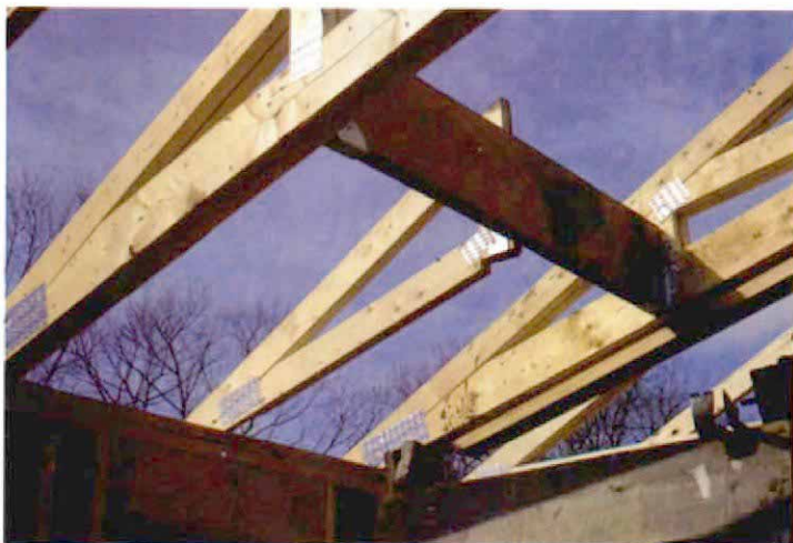
Wide skylights in truss roofs. A truss roof can be engineered to accept a wide skylight. Here, trusses have been doubled, and a small monotruss that fills in the roof below the skylight hangs on a header.
