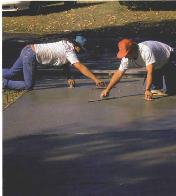
A special tool cuts the contraction joints. Contraction joints score the slab so that cracking from the curing process occurs at these points rather than at random.
