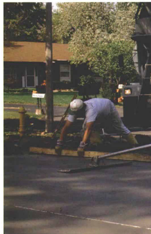
Screeding cuts concrete to the right height. A long, straight 2x4 or aluminum box beam is pulled across the surface of the concrete while it is moved in a side-to-side motion. Screeding brings the level of the concrete down to the top of the forms and consolidates it at the same time.
