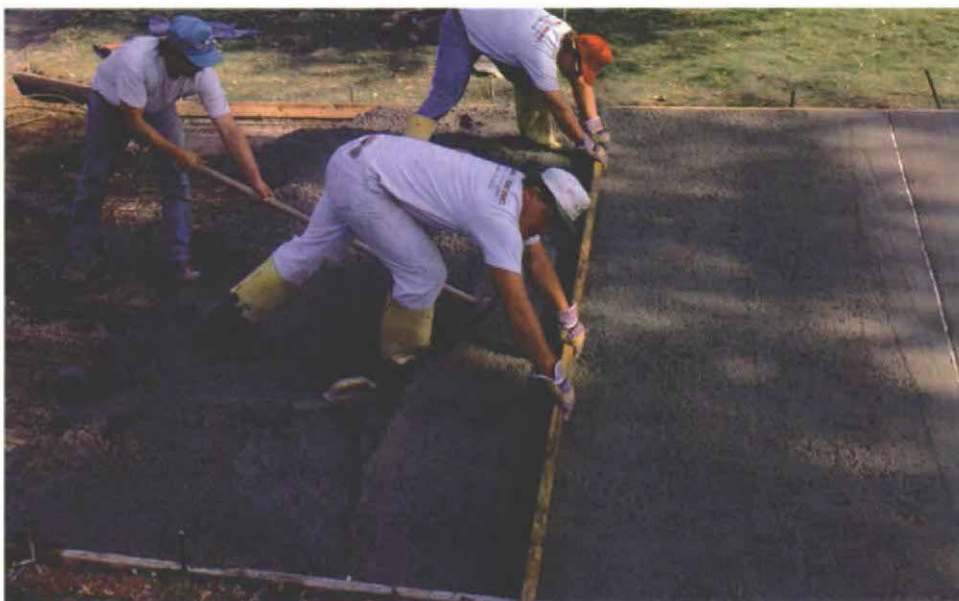
Screeding cuts concrete to the right height. A long, straight 2x4 or aluminum box beam is pulled across the surface of the concrete while it is moved in a side-to-side motion. Screeding brings the level of the concrete down to the top of the forms and consolidates it at the same time.
