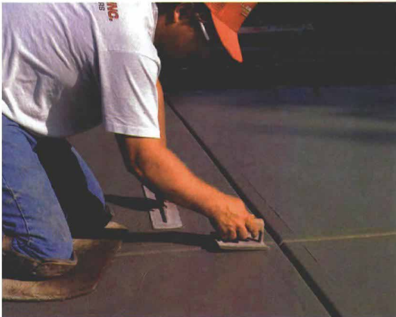
A special tool cuts the contraction joints. Contraction joints score the slab so that cracking from the curing process occurs at these points rather than at random.
