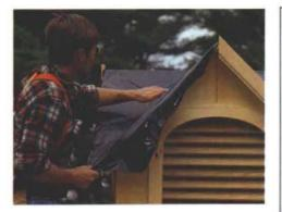
**Blocking the elements.** This cupola's roof was covered with a bituminous rubberized roof undercoating and then cedar shingles.
