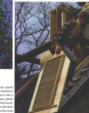
**Cheaper than a crane.** After building the top section of the cupola on the ground in his shop, the author had to haul each prefabricated piece carefully to the peak of his boat-barn roof for reassembly. He found that some sanding and cutting had to be done during assembly.
