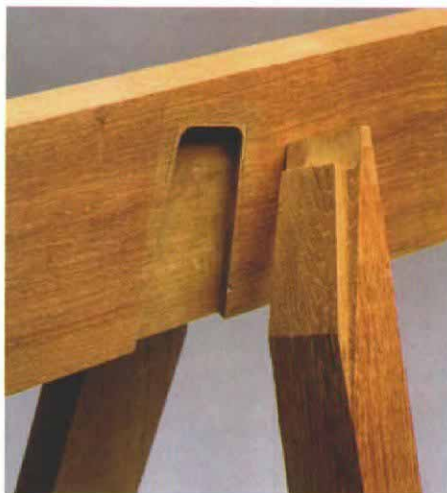
An elegant connection. Although it can be tricky to cut, a tapered sliding dovetail makes a strong and detachable joint between the leg and the cross beam.
