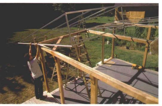
**It's sturdy and lightweight, but it's bulky.** Although the two sections of awning frame for the author's porch weigh only about 50 lb. apiece, they are unwieldy because of their size. One person can handle the frame, but it works better with two people on the job. If the frame had been in three sections instead of two, another beam would have been necessary.
