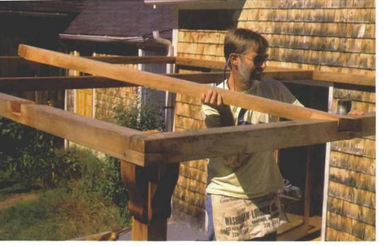
**Diagonals and center beam ensure strength.** Although it doesn't have to carry a great deal of weight, the seasonal-porch structure does have to be sturdy enough to hold the awning down during high winds and to last through many knockdowns and installations. The author used diagonal beams to brace at outside corners of the top plate and a center beam for added stability.
