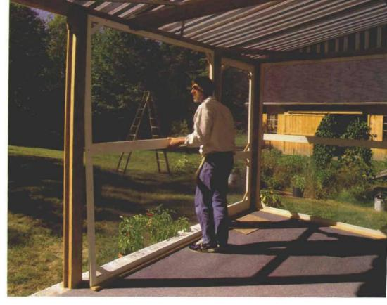
**Big screens need extra bracing and support.** Wide screen stock and comer brackets prevent bulging screens, which are further stiffened when the screens are screwed into place. The cedar sill at the bottom of the screen holds down the carpeting and keeps water from the frame.
