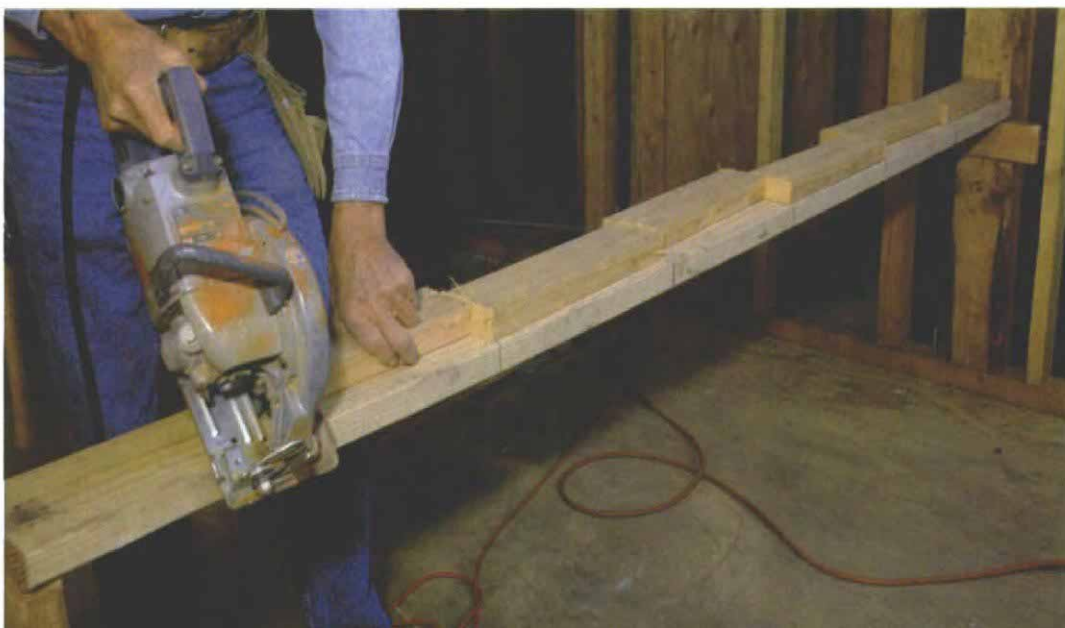
Cutting blocking is quicker with a graduated bench. One method the author uses to cut blocking is to build a simple bench from dimension lumber, supporting one end from an interior partition wall and propping up the other. The blocking is cut by sitting along marks made across the bench every 14½in.
