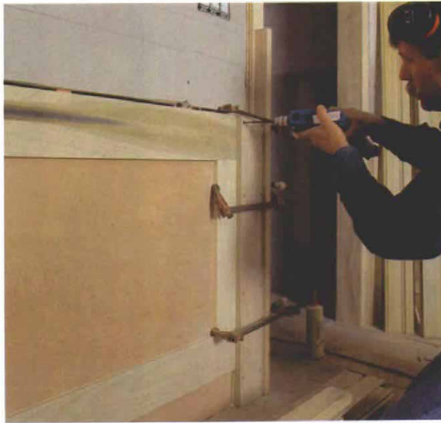
The panels end at pilasters. At each door opening, a pilaster the same height as the paneling is glued and screwed to the plywood substrate and to the flat subcasing attached at a right angle to the jamb.
