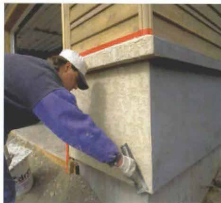
One worker should trowel the finish coat. To ensure a uniform appearance, the same person should trowel the final coat of stucco. On big jobs one worker can apply the finish while a second worker textures it.
