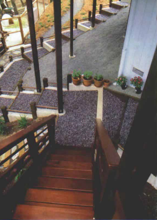
Pathway as retaining wall. Stepped concrete grade beams under the deck create a terrace of steps that help to stabilize the hillside. Photo taken at 6 on floor plan.
