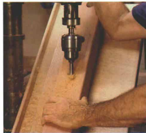
Fabricating posts. With the post fixed at the correct angle, mortises for the 1-in. copper pipe rails were bored with a 1½-in. Forstner bit.
