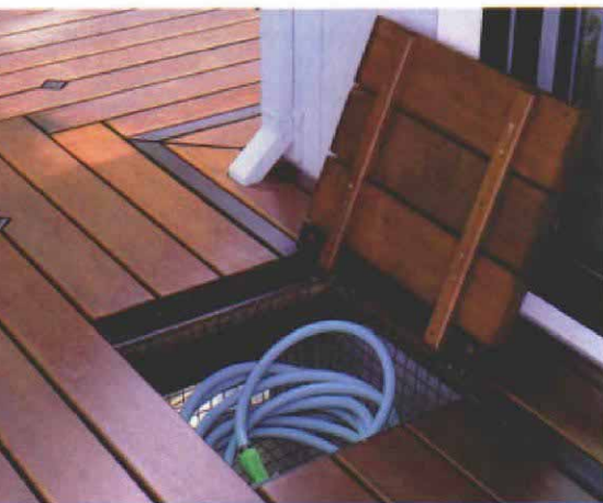
Housing the garden hose. A wire basket topped with a trap door conceals the hose. Behind it, a band of ebonized redwood borders the deck. Photo taken at C on floor plan.
