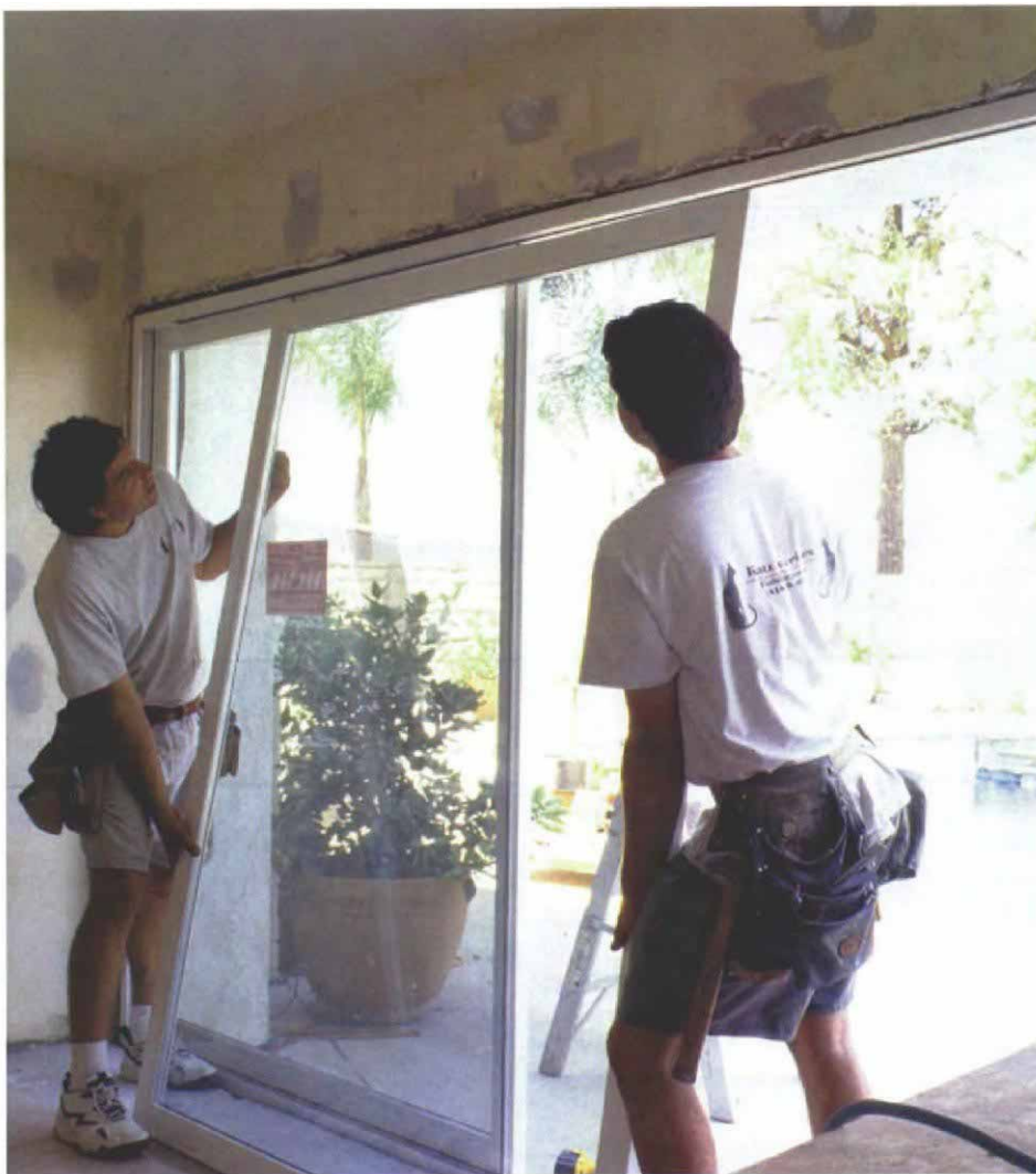
Most panels go in top first. The door panels are installed after the frame is secure in its opening. Most door panels slip into a channel in the head jamb first; then the bottom edge is set down over the track on the sill.
