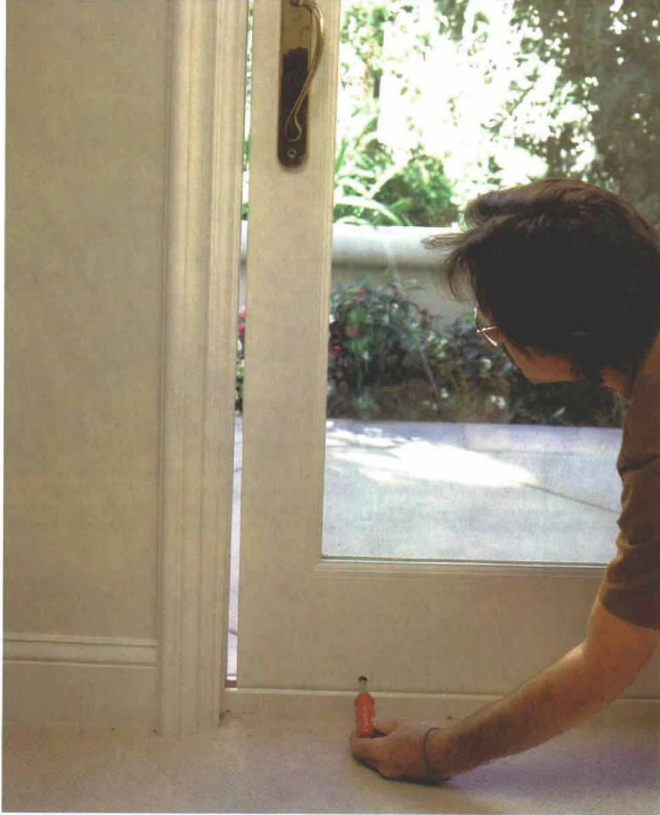
Tuning the sliding panel. A screw is turned to raise or lower the wheel, which brings the edge of the sliding panel parallel to the jamb.
