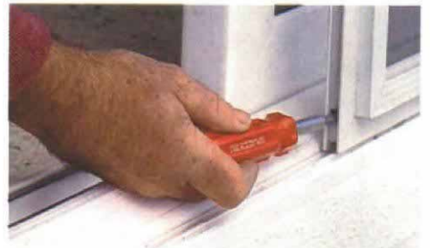
Screws adjust the screen wheels. Screws in the edges of the screen adjust the height of the spring-loaded wheel as well as the tension on the springs to keep the screen from binding.
