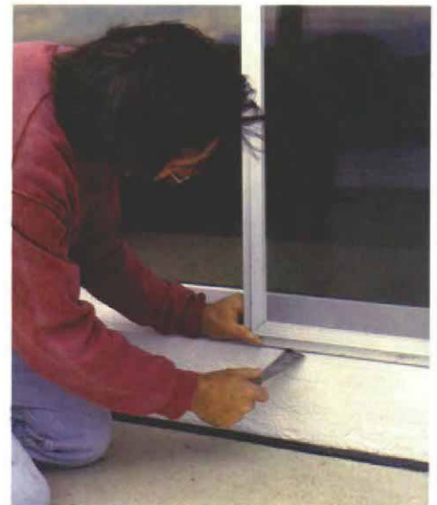
A putty knife puts screen wheels on track. If the screen panel rides on spring-loaded wheels, a stiff putty knife can be used to depress the wheel and guide it onto its track.
