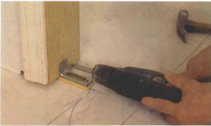
12. Align jamb brackets with the door track. At the base of each side jamb, an L-shaped bracket supports a pivot pin mounted in the bottom of the pivot door. The serrations in the slot capture the star-shaped pivot pin at the bottom of the door, holding it at the desired distance from the jamb. The bracket sits atop a \frac{3}{8} -in. thick plywood block, which keeps the bracket from being buried by the carpeting. A pencil mark on the side jamb notes the centerline of the door track above.
