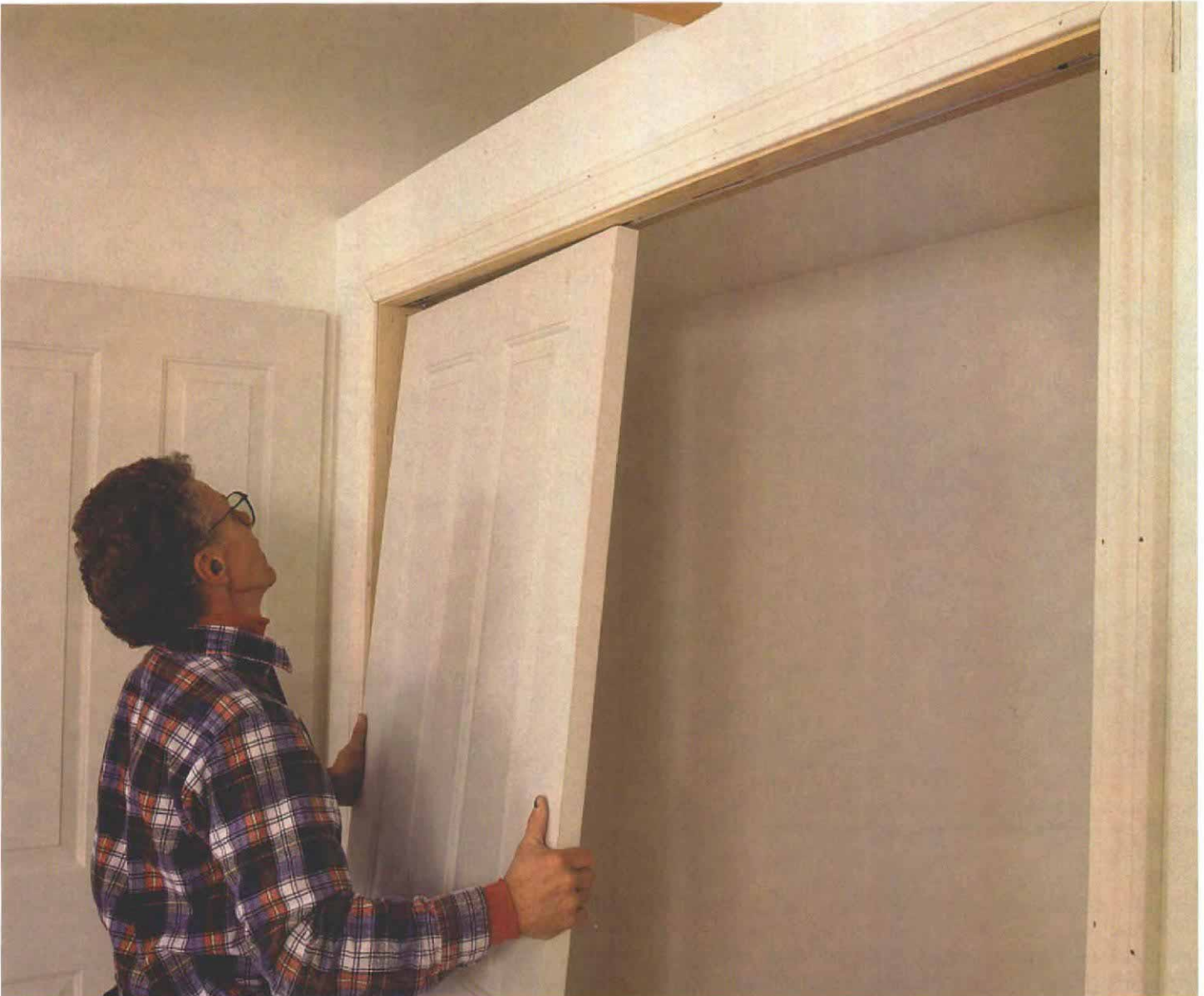
15. Install the doors from the top. Insert the top pivot pins into their slots, and push up to compress the springs. This makes room for the lower pivot to clear the jamb bracket as its pin is located in the serrated slot.
