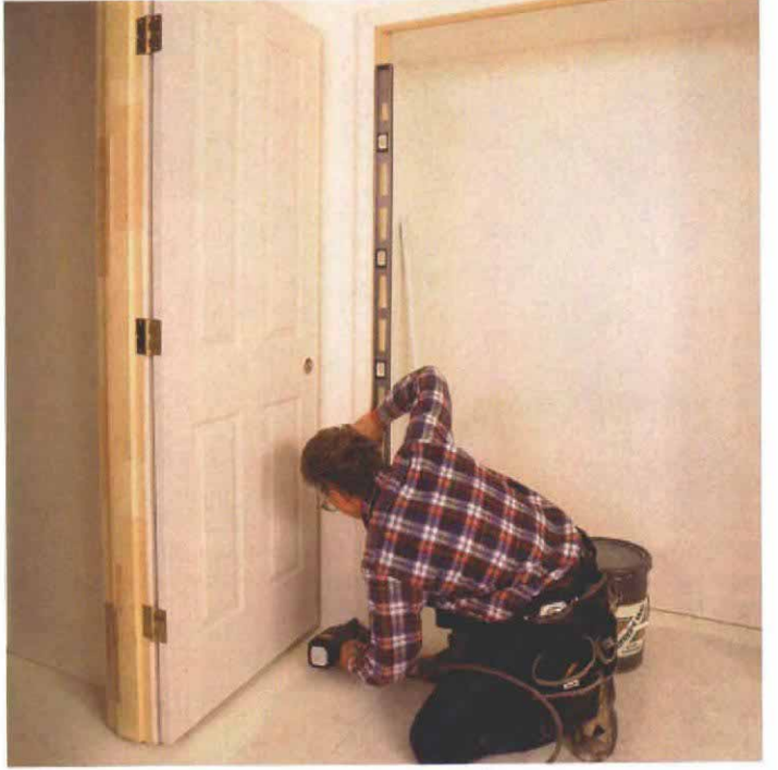
7. Plumb the side jamb. Britton uses the 6-ft. level to check the side jamb for plumb, moving the bottom of the jamb toward or away from the trimmer until the bubble is centered. Once he's got it right, he affixes the casing to the trimmer with a nail near the bottom of the jamb.
