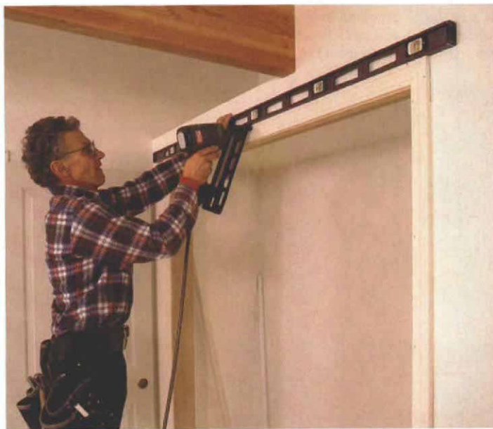
10. The head casing gets nailed on last. Britton takes a slight bow out of the head casing by flattening it against the level as he nails the casing to the header.
