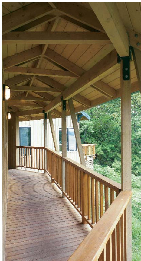
Planned for minimal disturbance. The bridge footings were kept to a minimum to avoid damaging sensitive tree roots. Photo taken at C on floor plan.
