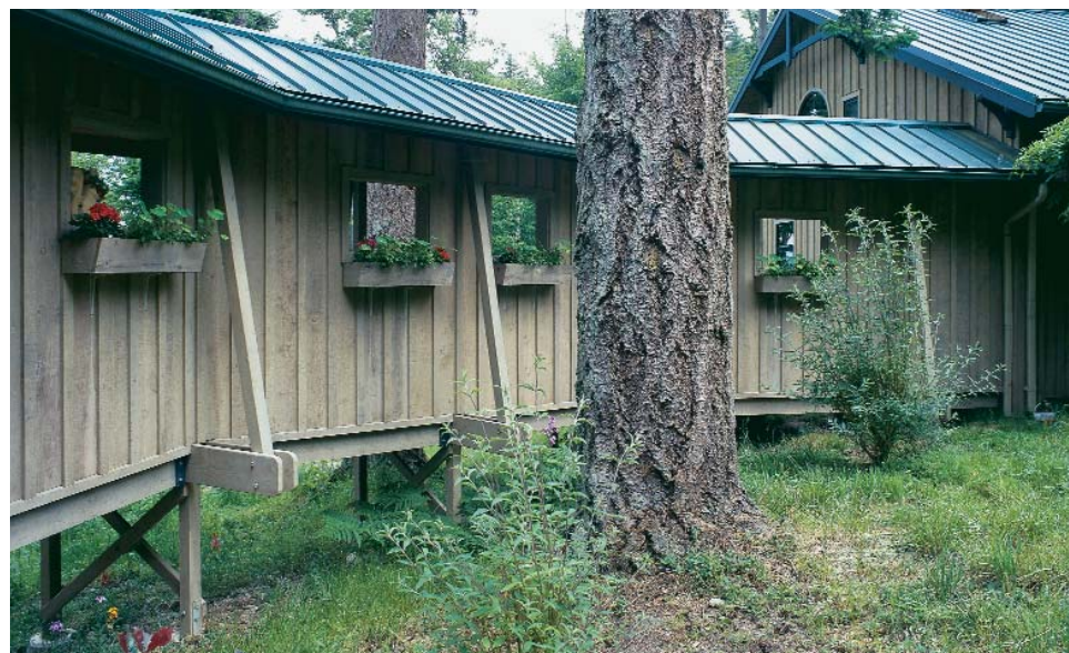
Planned for minimal disturbance. The bridge footings were kept to a minimum to avoid damaging sensitive tree roots. Photo taken at C on floor plan.
