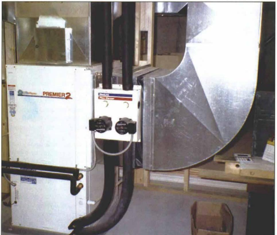
**A curve is more efficient than a 90° turn.** Air moves more efficiently through the large curve in this return duct than it would have if the installers had used a right-angle, or squared-off, fitting to bring air back to the heating unit.
