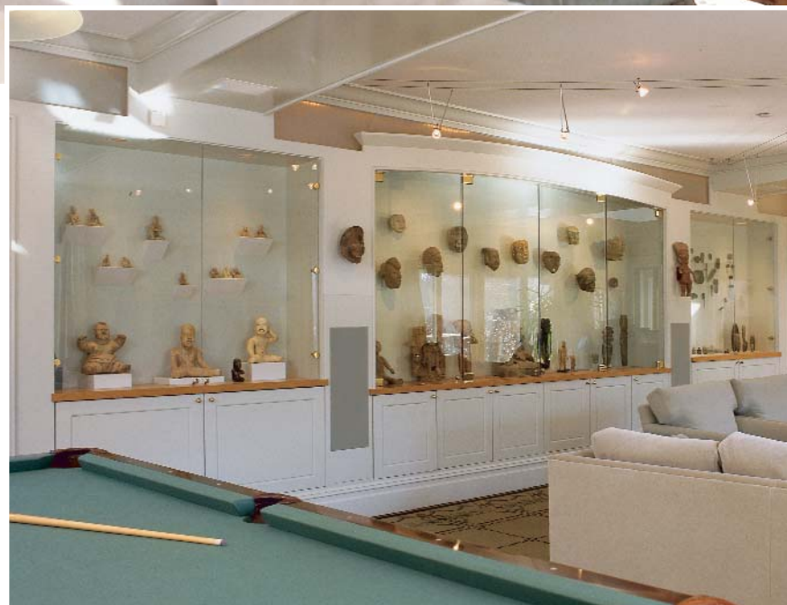
Recessed built-ins don't seem to rob space from the room. A secondary wall of MDF around this living room allows the display cases, cabinets, drapery pockets and valances to be recessed. The varying depth of the recess is revealed at the doorways.
