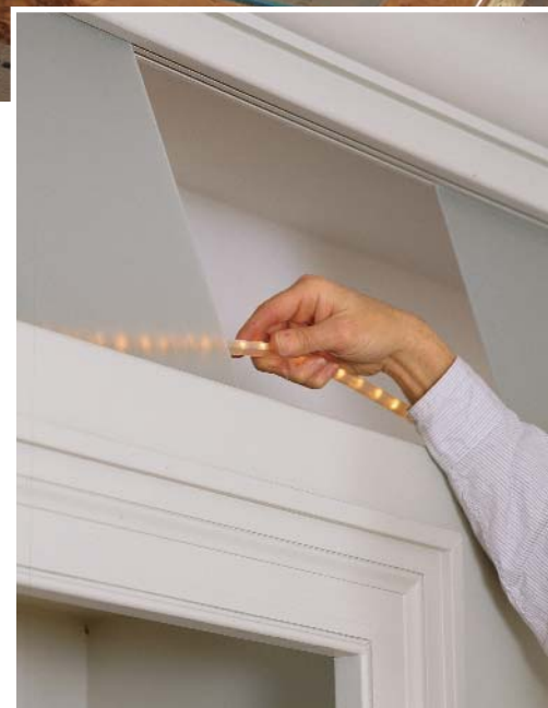
Flexible lighting is easy to install. Sliding-glass panels circle above the living room's built-ins. Routed inside, strings of tiny incandescent lights in flexible tubes create a warm glow.
