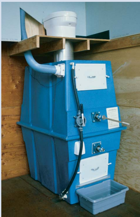
A standard composting toilet. In the Phoenix system, a conventional composting toilet must be installed directly above the basement composting unit. Another type of toilet, the foam flush, can be installed at an angle away from the basement unit. Photo courtesy of Advanced Composting Systems.
