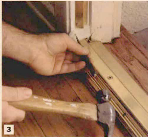
3 Corner pads complete the seal. Corner pads are the best insurance against light and air penetration at the bottom of a door.
