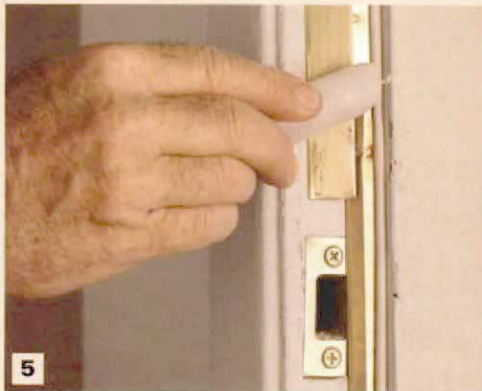
5 Waxed and ready to fight the weather. Paraffin wax silences the strip and ensures smooth door operation.
