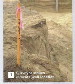
Stakes are driven at the ends of the first wall.
