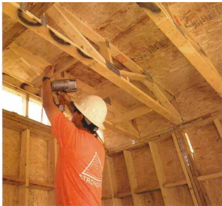
Blocking supports soffits that run parallel to the ceiling joists. The soffit's top plate is then nailed to the blocking. Horizontal blocks between the studs slow the spread of fire to the soffit and the floor above.
