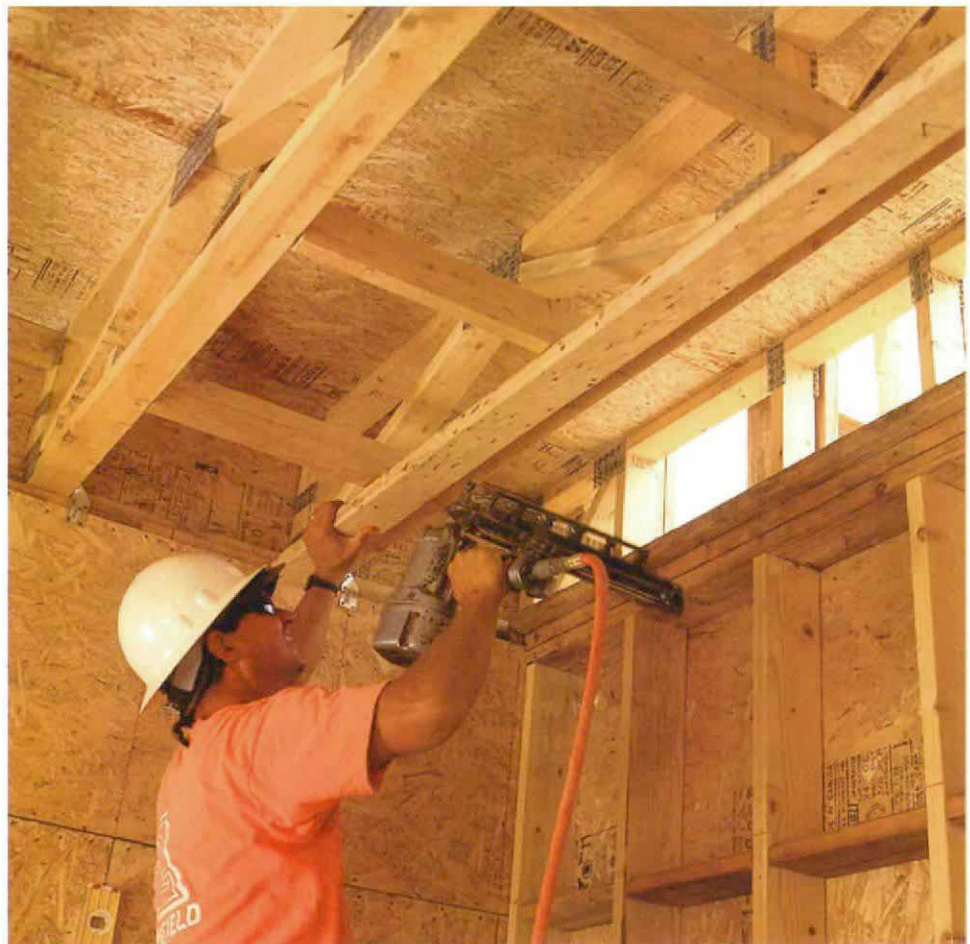
Blocking supports soffits that run parallel to the ceiling joists. The soffit's top plate is then nailed to the blocking. Horizontal blocks between the studs slow the spread of fire to the soffit and the floor above.
