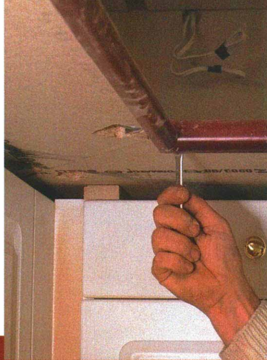
Tighten miters at the front first. To assemble a miter, align the front edge and gently tighten the front bolt. Then insert a bolt in the rear mortise, line up the joint, and insert the remaining bolts.
