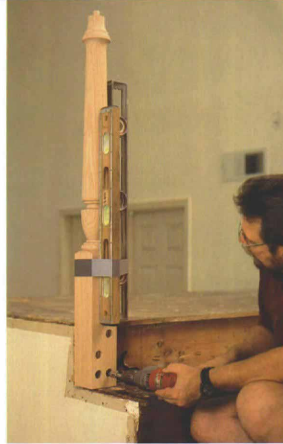
Landing newel is bolted to both riser and tread. Unlike the starting newel, the landing newel is bolted in two directions. The lower left hole provides access to the vertical hanger bolt; lag bolts are driven horizontally into the other three holes.
