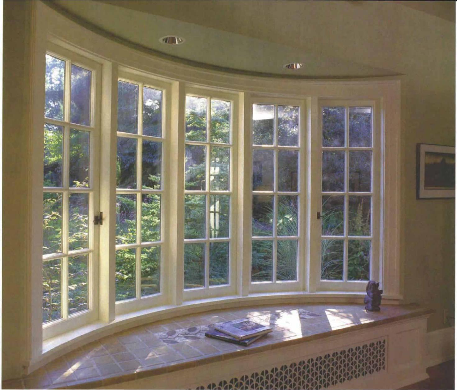
Douglas fir that had been resawn from 1x and 2x material. After planing down individual plies, I glued them together with plastic resin glue, rolling it onto both surfaces with a fine-nap paint roller 4 in. wide. Plastic resin glue has a long open time, so you don't have to hurry as with yellow glue. Depending on which piece of trim I was gluing up, either the inside or outside surface of the curved header made a good bending form. It took just about every clamp I owned.
