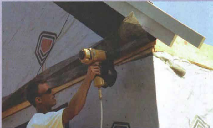
Tying the gable to the house. Once the gable is braced in position, the bottom plate is nailed off (top photo), and the sheathing that was left overhanging is nailed to the house framing (bottom photo).
