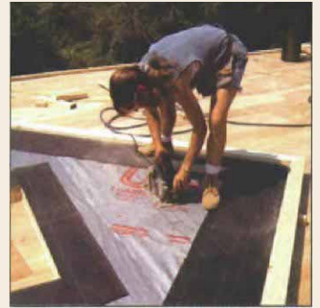
A hole for air but not water. A bow vent begins with a hole cut in the wall properly sized for the area to be vented.
