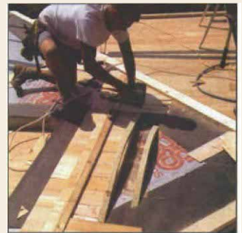
The bow is framed with 2xs. Beveled nailers are attached above and below the vent opening.
