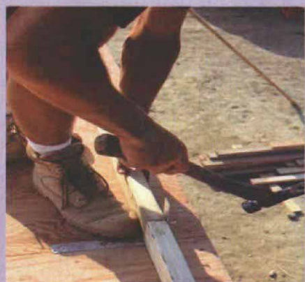
Metal straps act as wall hinges. Nailed to the floor framing and then to the bottom plates, straps keep the wall from slipping off the deck's edge.
