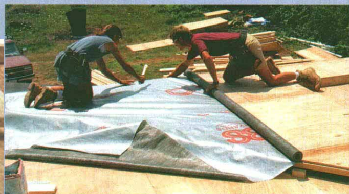
Gift-wrapped gable. With the wall lying flat, the housewrap can be stretched out and stapled without wrinkles.
