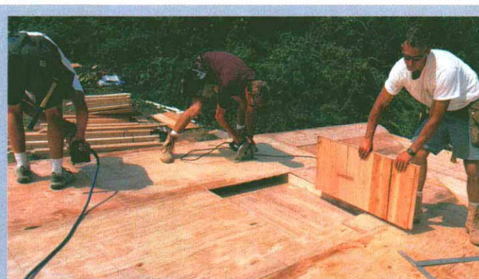
It sure beats carrying plywood up an extension ladder. Sheathing the gable wall while it's flat means that sheathing doesn't have to be held in place while it's being nailed. Cutting and nailing also go much quicker horizontally.
