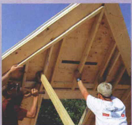
Braces help with the lift. With the wall held in place at about a 45° angle, 2x braces are nailed high up on the studs (photo above). The braces then help to control the final push (photo right) and finally are nailed to blocks attached to the floor framing.
