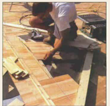
Shingles follow the line of the bow. Shingles are nailed to the nailers using a stretched string as a guide.
