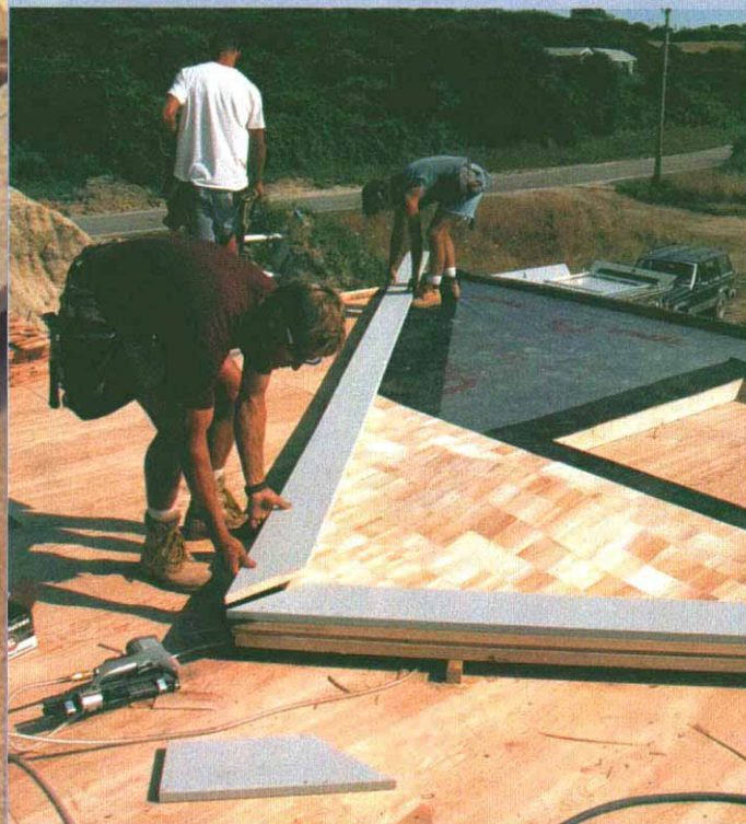
Fitting gable trim in comfort. Instead of working off tall ladders or awkward staging to get all the trim cuts right, the author fits all the trim perfectly with the wall lying flat.
