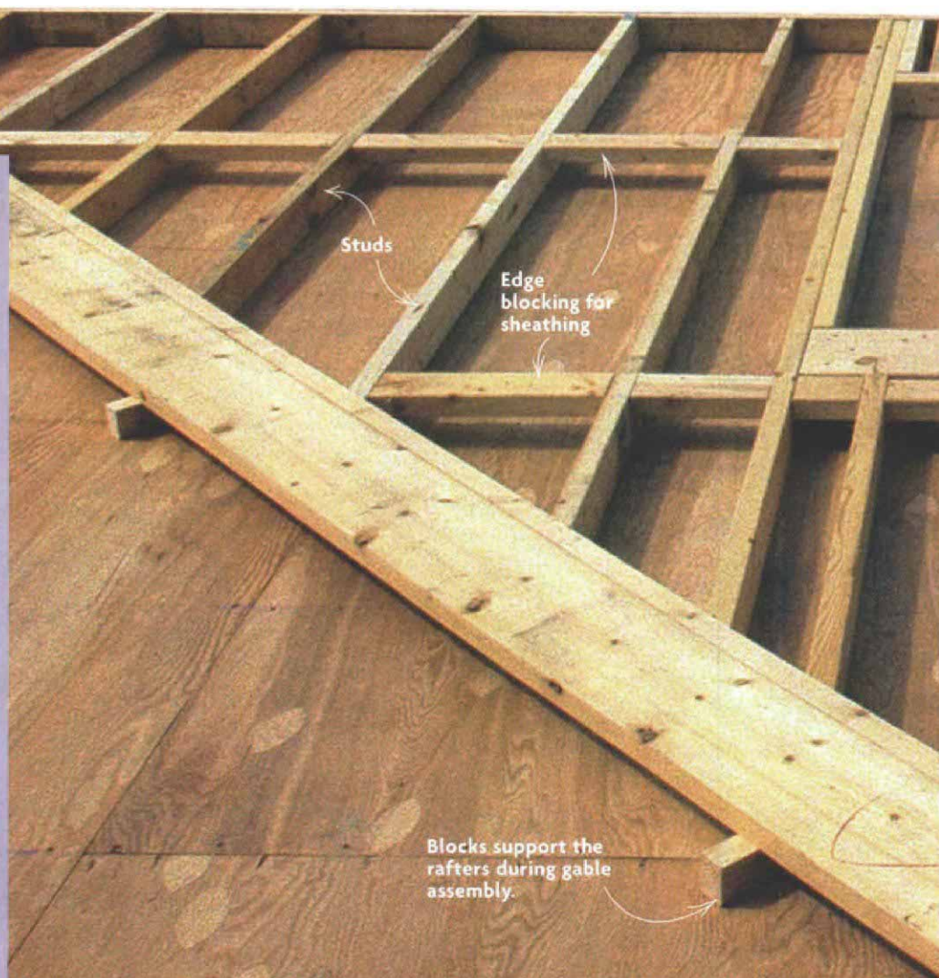
Blocks keep the plates straight. Top plates are tacked to 2x blocks that have been ripped to 2 in. The blocks will also support the gable rafters.
