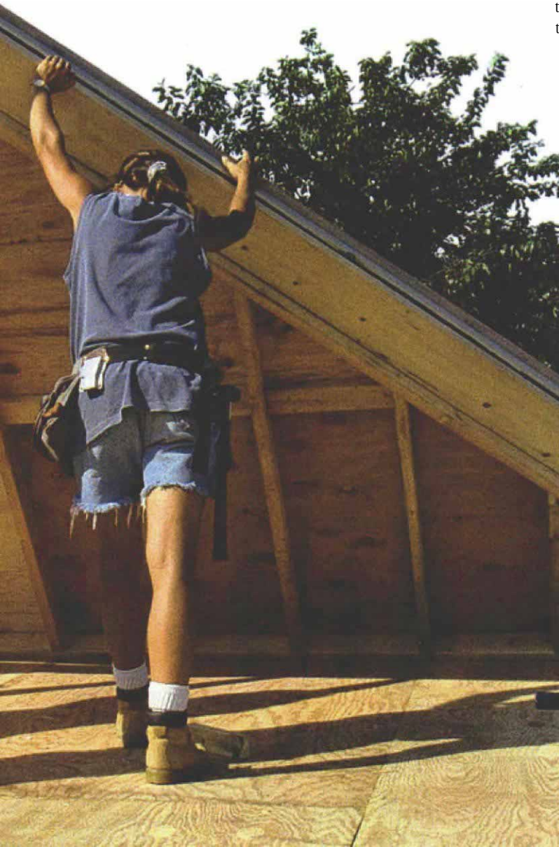
Finding the peak. The first step is laying out the upper plates and snapping chalklines for other framing details.
