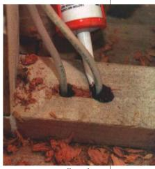
Intumescent caulk makes a fireproof seal. Holes between floors are potential flues for fire and must be sealed. If fire melts the insulation or pipe, the caulk expands and forms a fire-stop.
