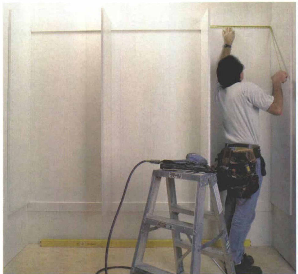
The only measurement in the closet. Other than the initial measurement for the ledger, the only measurement that needs to be taken is for the width of the remaining space. All other measurements are predetermined.
