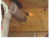
Holes and gaps in the framing pass lots of moisture. Sealing the holes is simple, though. A shot of urethane foam stops the flow of moisture-laden air.
