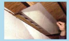
A mirror reveals open block cores, a great moisture source. The fix is easy, though. Cap the cores with expanding foam or simply stuff them with wads of plastic sheet.
