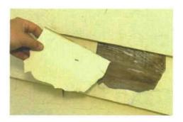
Peeling paint is a symptom of moisture trouble. Interior moisture, driven outward by air pressure, condenses in cold walls. Diffusing through the siding, the water makes paint peel.
