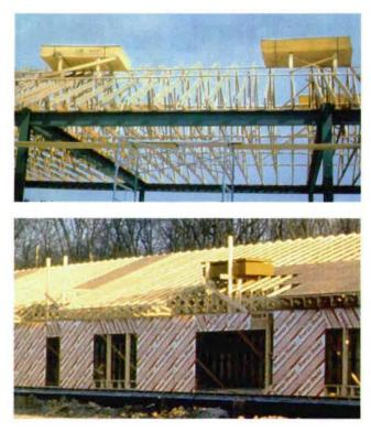
The bracing for the top chord is typically satisfied when the roof sheathing is applied. The bottom-chord bracing is normally accomplished by placing a row of 2x4s on top of the bottom chord and then running them alongside a panel point (the point where the webs and the bottom chord meet) for the full length of the building. In a wide building, these bottom-chord braces should be roughly 10 ft. o.c.
