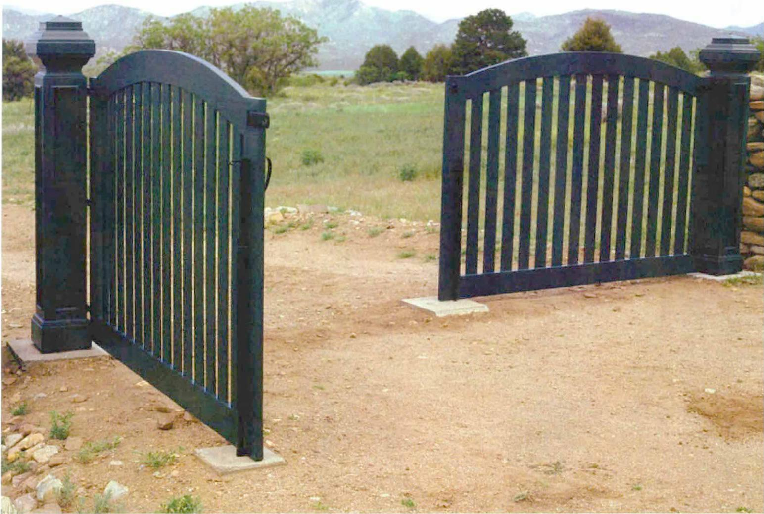
**A fully supported gate.** With their free-swinging ends resting on concrete pads when they're open and when they're closed, these gates have to carry their own weight only when they're swinging (photo above). To bolster the gate against high winds, whether open or closed, 5-ft. long steel rods descend half their length into the concrete pads.
